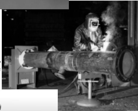
Pipe Shop Applications
